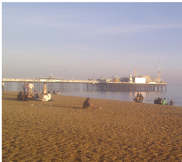
Brighton's Palace Pier
