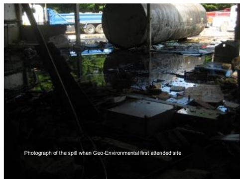
It was evident that contrary to the approved Method Statement, an attempt was made to move the tank without first removing the oil and making the tank safe for removal. Instead the brick cradle supporting the tank was broken out and some attempt was made to move the tank whilst still containing oil.
