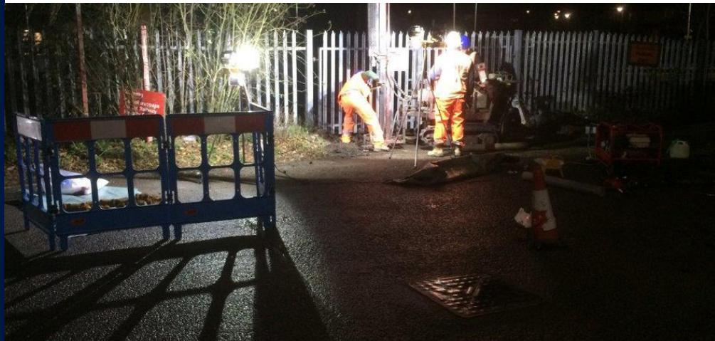
The Woburn Sands Formation was found to be medium dense, providing a moderate bearing pressure. However, in the event that conventional foundations may not be suitable, e.g. due to high structural loads (e.g. beneath the proposed foot bridge deck's support columns), an alternative such as piled foundations would be considered suitable.
