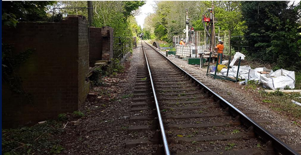
Classification of the embankment material, in geotechnical terms, was also required as this was to inform the stability of the slopes and the dimensions of the proposed wing walls.
